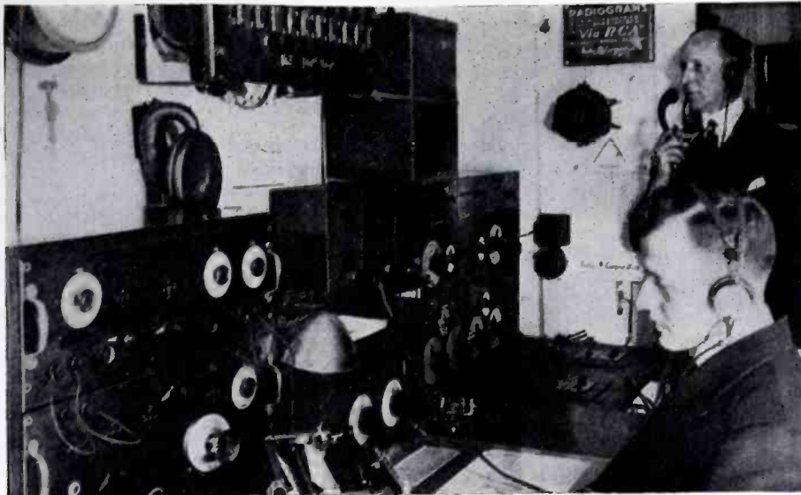
Ship installation—duplex set and radio room aboard the S.S. America with Harold G. Porter, Manager of the Pacific Division of the Radio Corporation of America, using the transmitter
