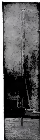
20 Ft. HERCULES Mast on roof.
