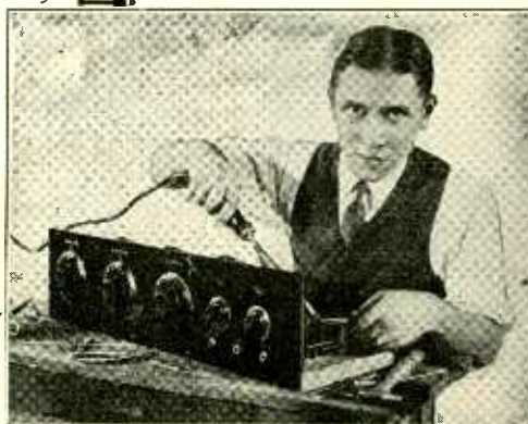
Front View KD-50 Neutrodyne Being Assembled
