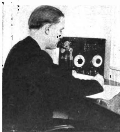
Transmitting department of the Chicago Board of Trade Station, KYW
