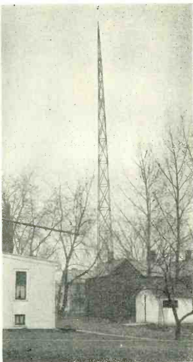
A vertical harp antenna and counterpoise is used at 8ZG station
