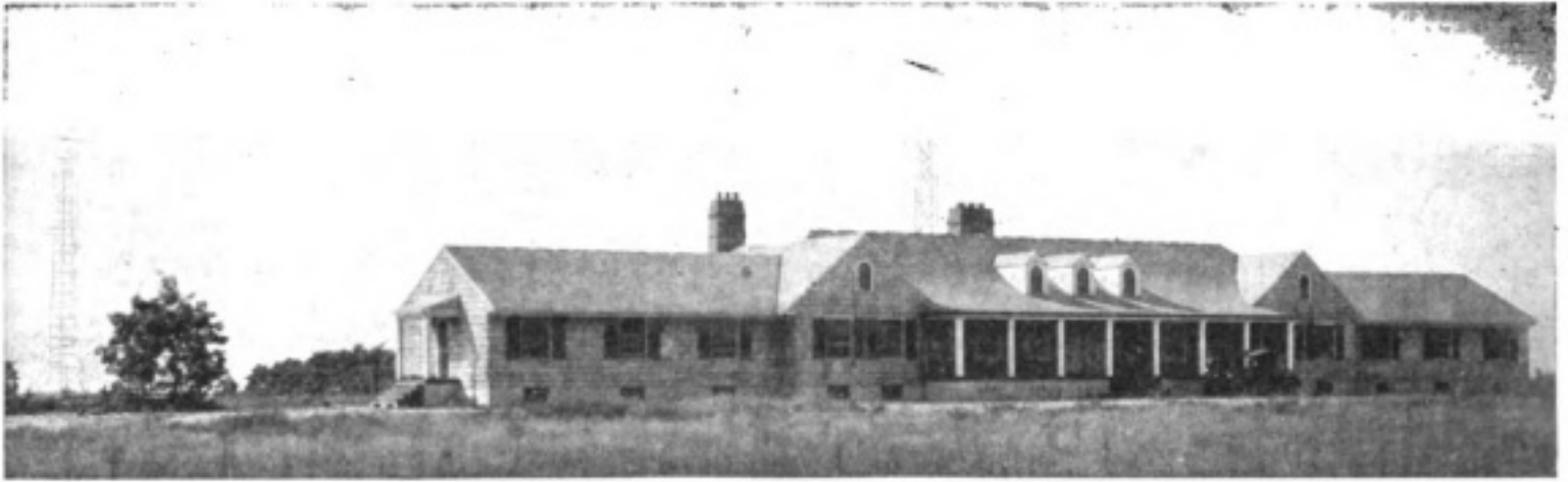
The Community House at Radio Central which accommodates the bachelors of the operating staff. Separate cottages are provided for the married personnel
