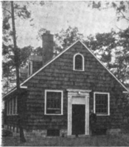
Multiplex receiving station located at Riverhead, L. I., sixteen miles east of Radio Central
