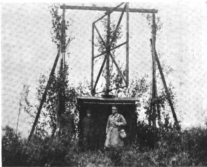
A camouflaged gonio, or wireless compass station of a type operated by the Radio Section (Intelligence) Signal Corps, in France
