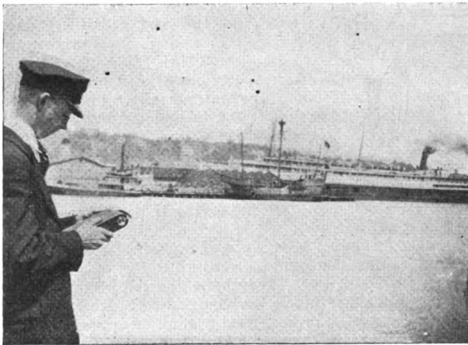
Evidence of the existence of the troublesome kodak that marred the early pleasures of two enthusiastic wireless operators
