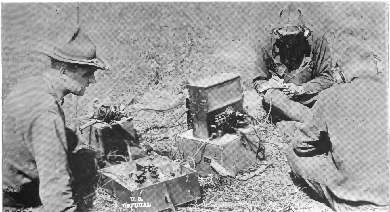
Receiving practice with an American made SCR 54 Receiver and a French Amplifier Type 3 ter
