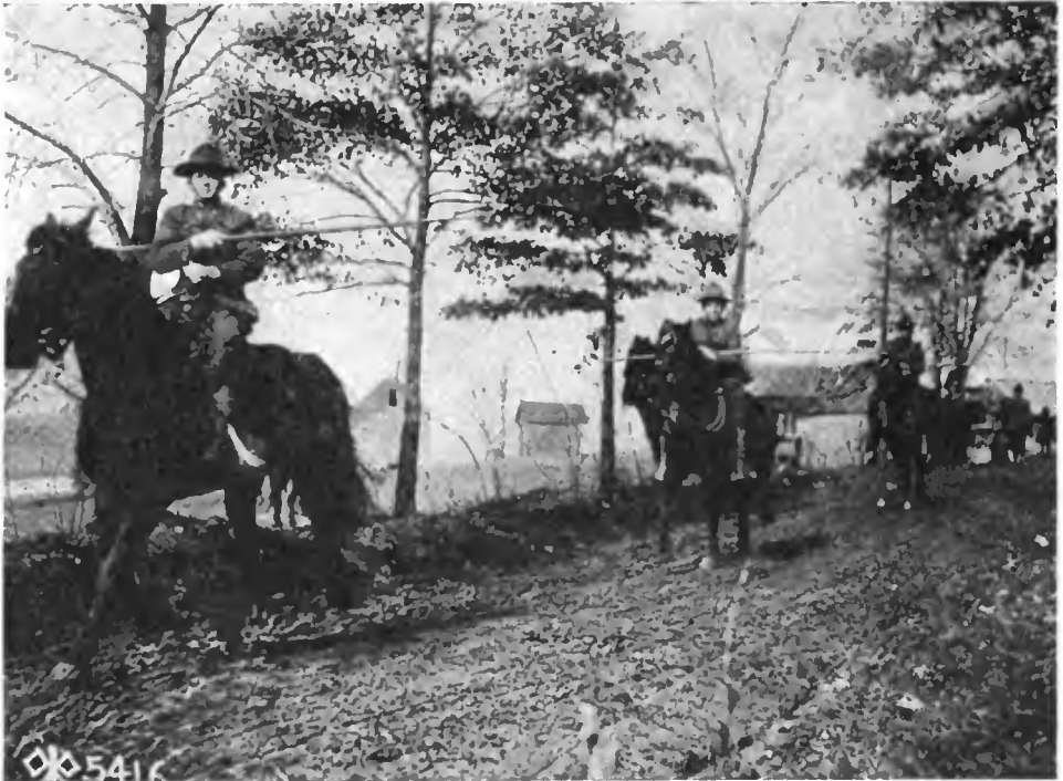
Signal Corps men laying the lines in accordance with the regulations prescribed in the accompanying article
