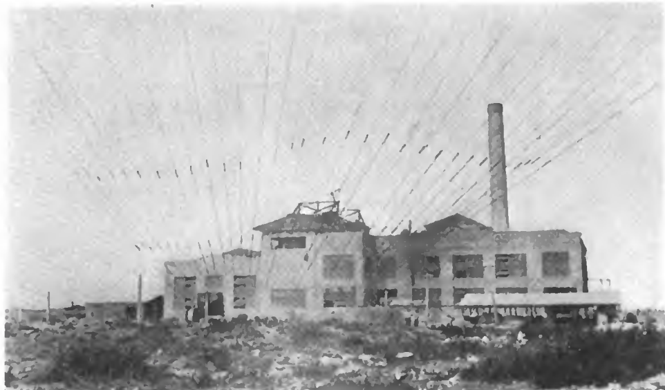
Typical power plant of a Marconi long-distance station, showing aerial wires leading in
