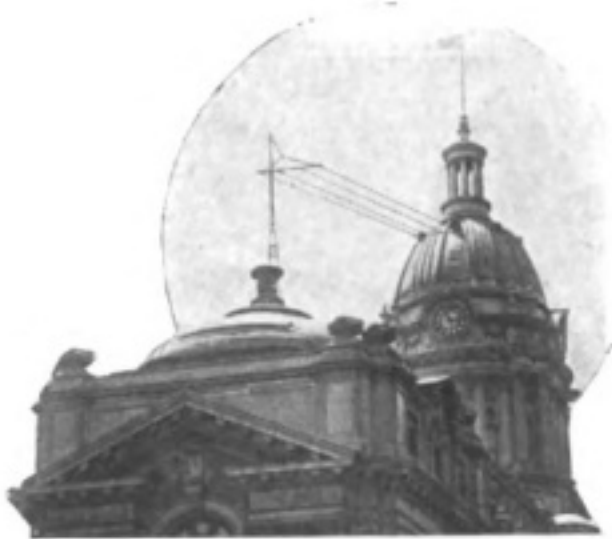
The aerial on the Headquarters building
