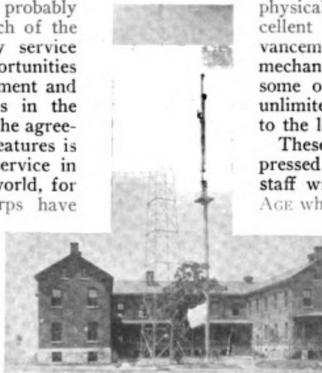
The old mast standing beside the new steel tower erected by enlisted men in the United States Army Signal Corps School at Bedloe's Island, New York
