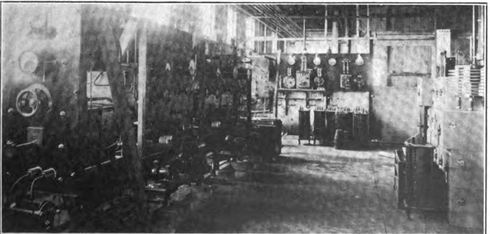
In this room all the apparatus is tested and inspected by a corps of experienced men.
