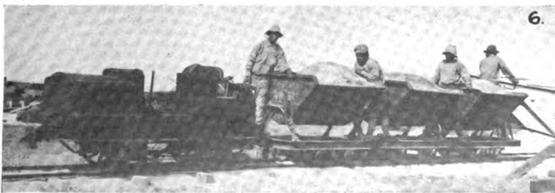
(4) One of the methods of transportation employed in delivering mast sections to the Honolulu sites. (5) Condenser pit excavations made under difficulties. (6) An illustration of the ingenuity of the Marconi engineers: the chassis of an automobile transformed into
