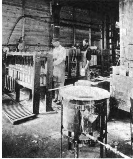
The Plating Room, where the Glass Condenser Jars are Copper-Plated Inside and Outside
