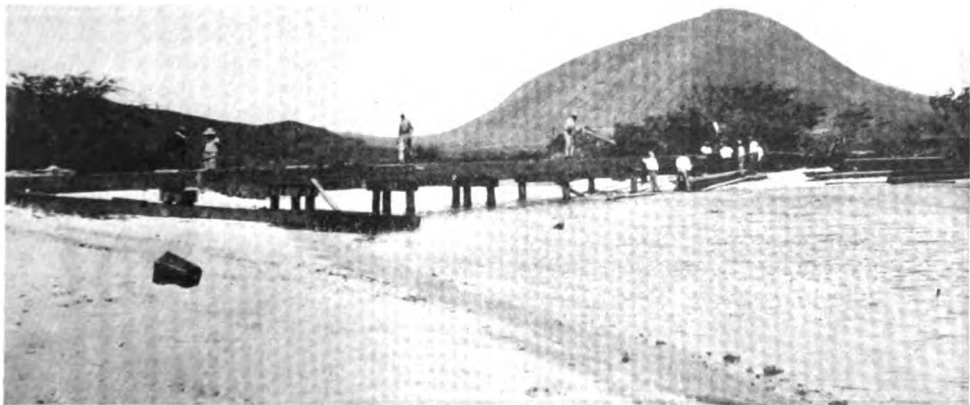
From disheartening experience transportation of materials to Koko Head by the sea route has proven neither safe nor speedy. Consequently the greater part of the material has been hauled to the site by road. When this was first tried in the midst of a tropical downpour the wagons slid sideways off the muddy roads and the material finally had to be brought piecemeal to its destination. The roads have been improved by regrading and the bridge shown in the photograph has been built across the pond.
