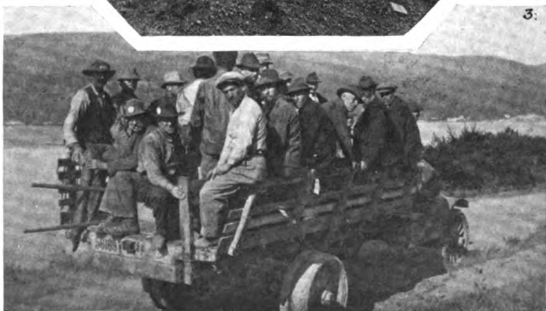
1. Distributing poles for the operating land line by which the receiving unit automatically controls the sending apparatus. 2. One of the masts for the Belmar station as it reached the half-way mark. Two others, or three out of the six, are now half completed. 3. A typical group of workmen en route to daily tasks. A number of motor trucks have been acquired by the Marconi Company for transporting labor and materials.
