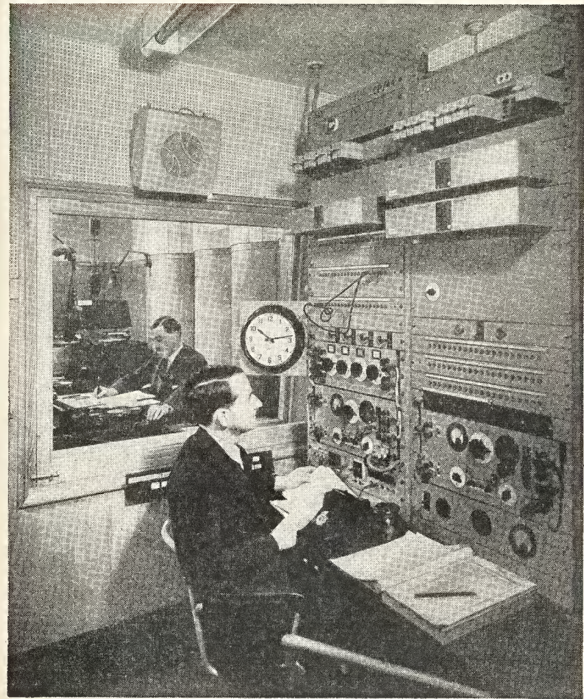
Control engineer in the Light Programme Continuity Suite. He selects the programme items, time signals and announcements in their proper turn. The continuity announcer can be seen through the communicating window.
