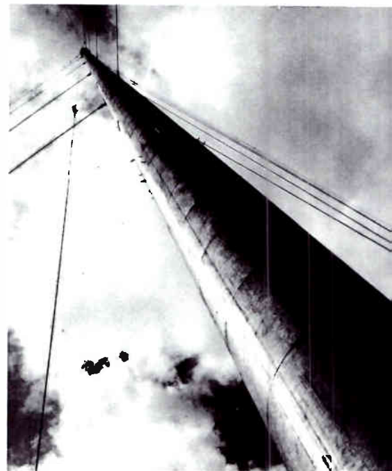
Nearly 1,300 ft of tubular steel, the Emley Moor mast which brought ITV to Yorkshire was the highest structure in Britain in 1956.
