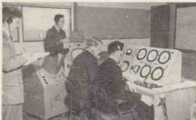
The control room, showing the Skipper (right) and Navigator (left) controlling a Jindivik during its airborne period through a series of push buttons. Telemetered information of the plane's height and speed is displayed to them on the five dials of the monitoring panel. Radar screen (right) indicates aircraft's position throughout the flight.
