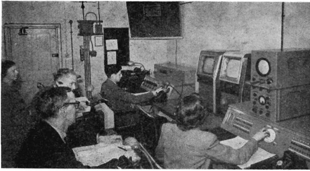
Fig. 7. The Central Control Room at Alexandra Palace
