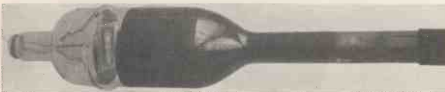
Photograph of Baird tube employed for producing still-picture signals.
