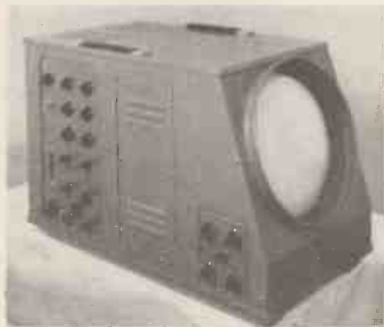
Fig. 1.—Cossor oscillograph with divided beam.
