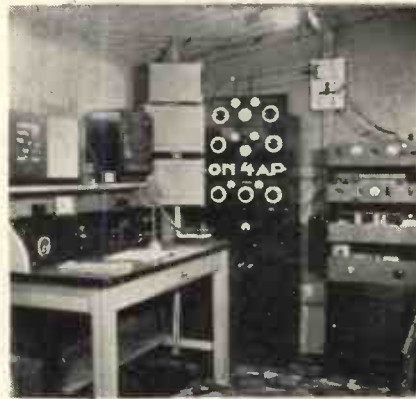
A typical European station is ON4AP, who is mainly interested in ultra-high frequency work. His 2.5 and 5-metre receiver and transmitter can be seen on the right of this photograph.
