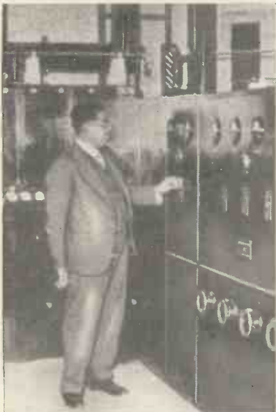
The amplifier and control room of the Eiffel Tower transmitter.
