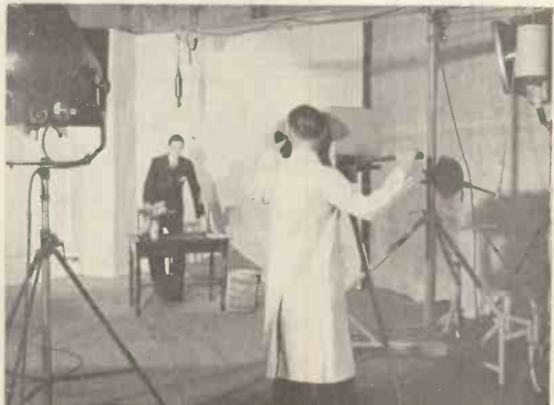
Scene in studio showing electron camera in operation on a three-quarter shot. Note the view finder for focusing the optical image on the cathode.
