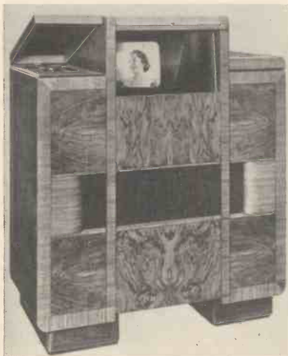
The photograph on the left shows the Marconiphone television receiver capable of receiving the Alexandra Palace sound and vision transmissions and also all broadcast sound. Model 702 (right) is for television and accompanying sound reception only.
