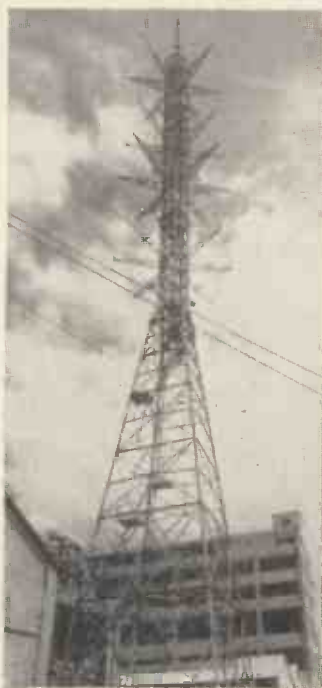
The 200 ft. high television aerial at Hayes.
