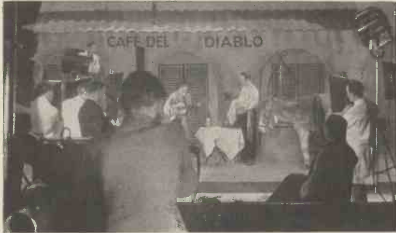
Almost every receiver will be in use when the programme includes a popular play. This is an actual scene during a transmission from the Baird studios at the Crystal Palace.
