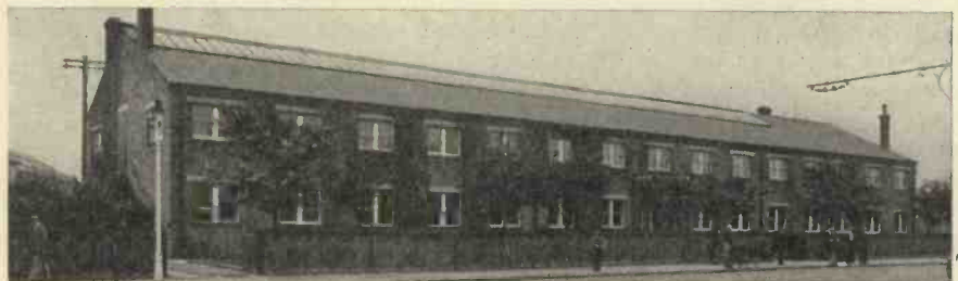
A photograph of the Plew Works at Waddon near Croydon.
