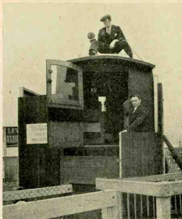
Transmitting apparatus in the caravan opposite the grandstand at Epsom. The announcer described the race from the roof.
