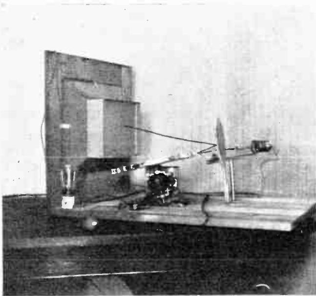
An interior view of Mr. Horst Hewel's home-made mirror drum vision apparatus. The ink line indicates the path of the light beam.
