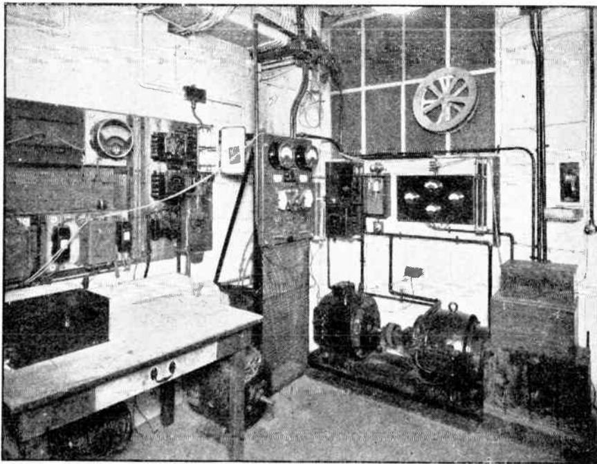
*Motor generating plant in the Baird laboratories. These machines furnish a 4,000-volt and 2,000-volt D.C. supply and a 230-volt A.C. supply.*
