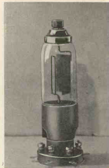
Typical example of photo-electric cells. Above is a gas-filled cell and on the right is the type used for "talkies."
