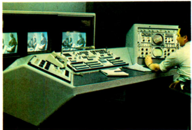
Control room at Croydon.
