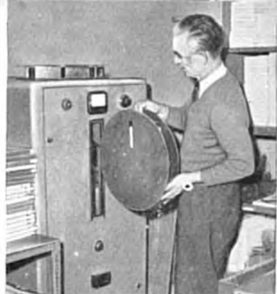
When Emitape returns from the studios to the BBC Central Maintenance Unit, it is re-serviced, passing through this 'washing machine'. A giant electro-magnet finally wipes off any signals remaining on the tape.
