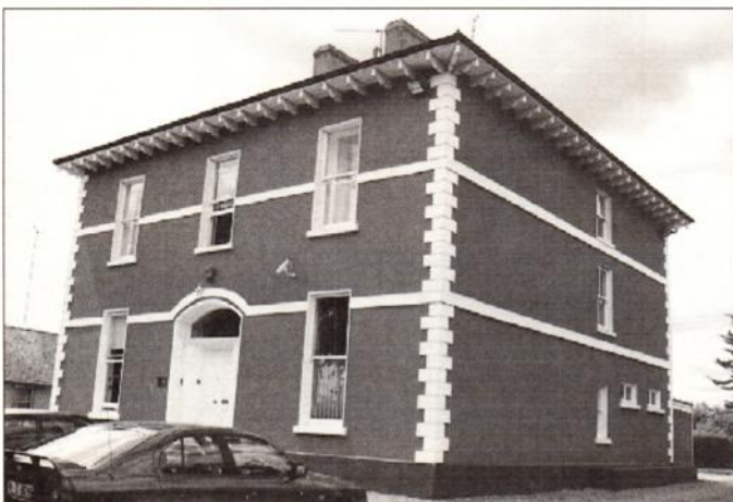
The magnificent Georgian building, 'Mornington House', home of the Atlantic 252 studio complex.
