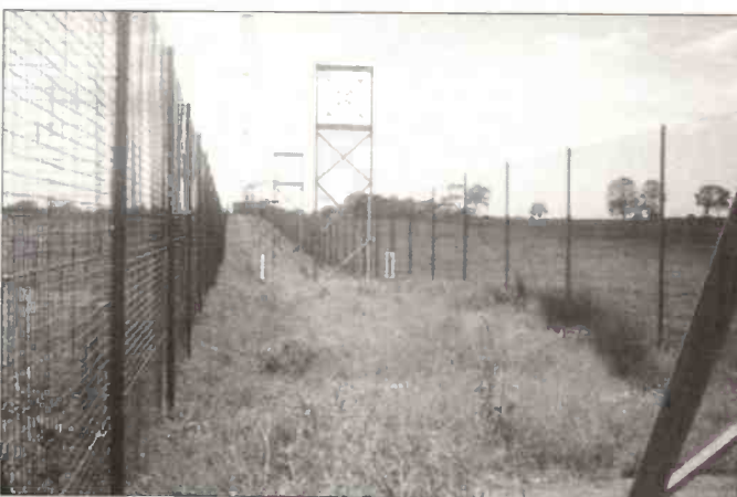
A shot of the overhead open wire transmission line. It runs some 250m and is 3m above ground. The impedance is 140 \Omega and has a loss of 0.4dB.
