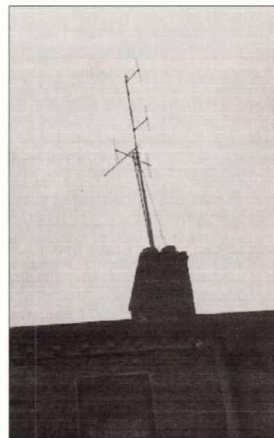
Radio Dublin's mast with v.h.f., m.w. and s.w. antennas stacked closely together.
