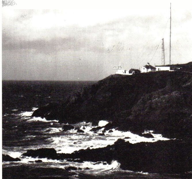
Portishead coast station. Photo courtesy British Telecommunications PLC.
