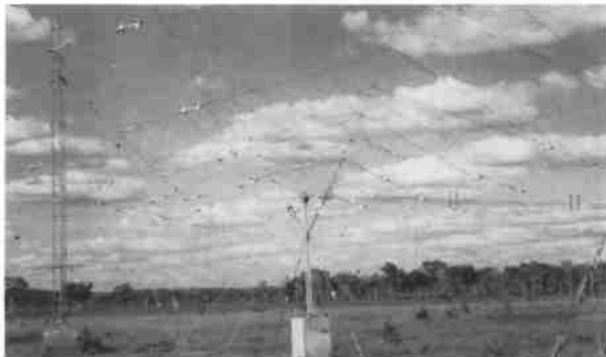
The antenna system at ABC's new Alice Springs station.
