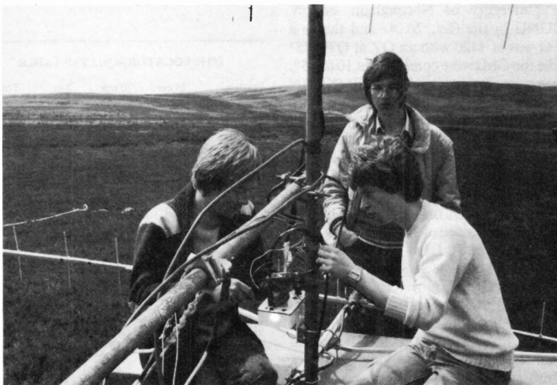
VHF NFD, 1981. Members of the Parallel Lines Contest Group checking out the 70cm. aerial system comprising four, 21 element Yagis. The box contains the GASFET preamplifier. The array went up and down five times before they were satisfied with its performance. Left to right are G8IMC, G8OBS and G8LYD. The location was 8 kms. west of Wrexham.
