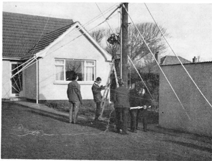
Raising a three-element Quad for 10-15-20 metres. On the right, the chaps doing the ground work, and on the left the job as finalised. This array, at the station of G3OFN (Redruth, Cornwall) is built up from 14ft. fibre-glassed bamboo, on a 2in. boom. It is finished in light blue, to match the sky—but even that does not camouflage it entirely!
