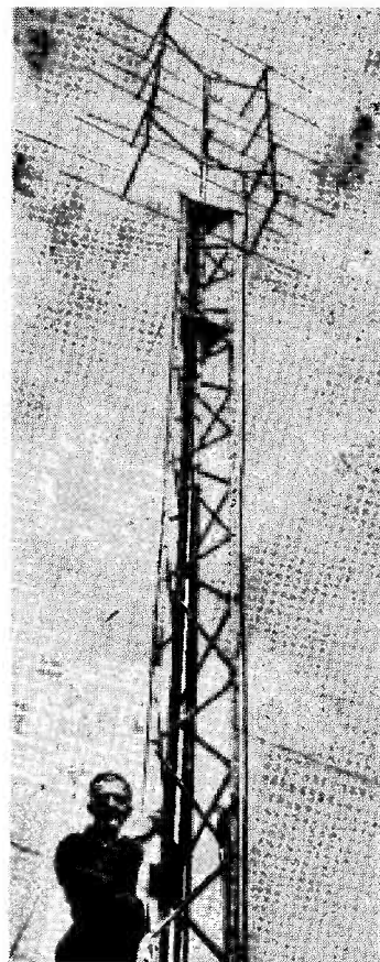
The 16-element stack at G4SA, Drayton, Berks., now at 48ft. Yes, that's Ted, holding on tight at the 24-foot rung.
