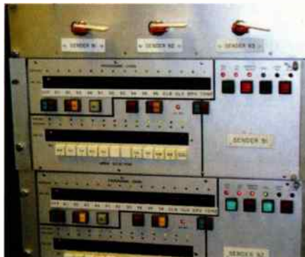
● (top) The delay sections that are switched in and out to create the slew effect.
