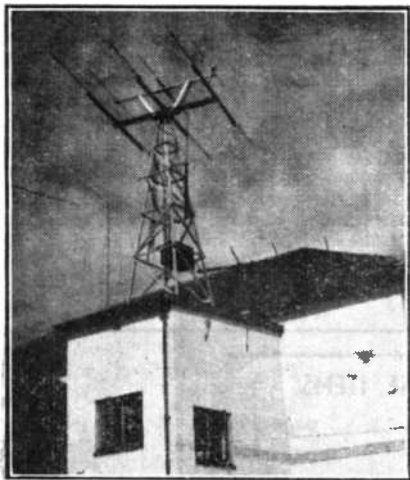
The other end — The 6m beam at ZSIP which recently pulled in PAoUM.
