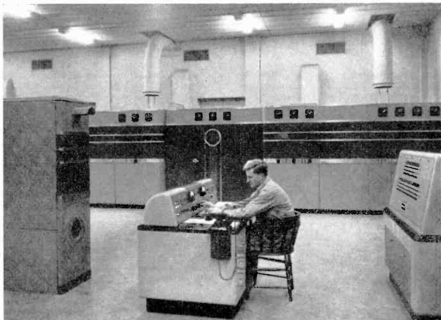
The 50 kW equipment of Radio Australia, V.L.C., at Shepparton, operating on various frequencies from 6 to 22 mc. There are 19 different directional aerial systems at this station, giving adequate coverage of all parts of the world at any time of the day.
