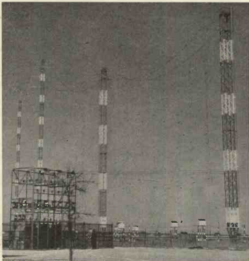
General view of the European aerial system of the Canadian Broadcasting Corporation ; two of the towers are 379 ft. high, one is 217 ft. and the fourth 165 ft. The aiming and reversing switches for the aerial curtains are remotely controlled from the transmitter building.
