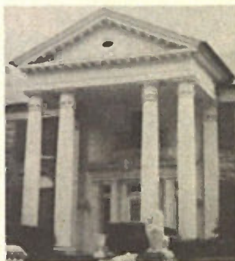
The entrance to El's home in Graceland.
