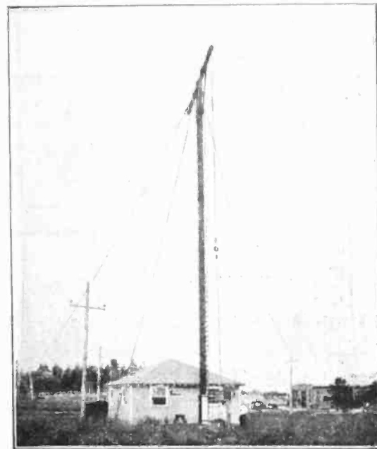
Vertical antenna used with the 32.79 meter transmitter illustrated below.
