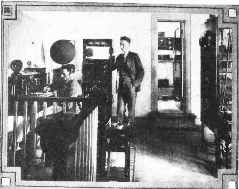
The control room and transmitter of the station.
