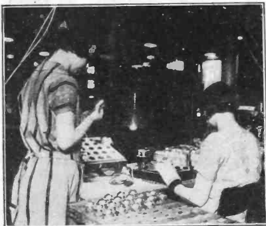
A batch of finished UV-201-A tubes undergoing the so-called jigger test, which means an electrical inspection for short-circuits, misplaced elements, broken or burnt-out filaments, and so on. The girl seated at the table attends to the jigger test, with a combination of lamps which tell-tales on defective tubes.
