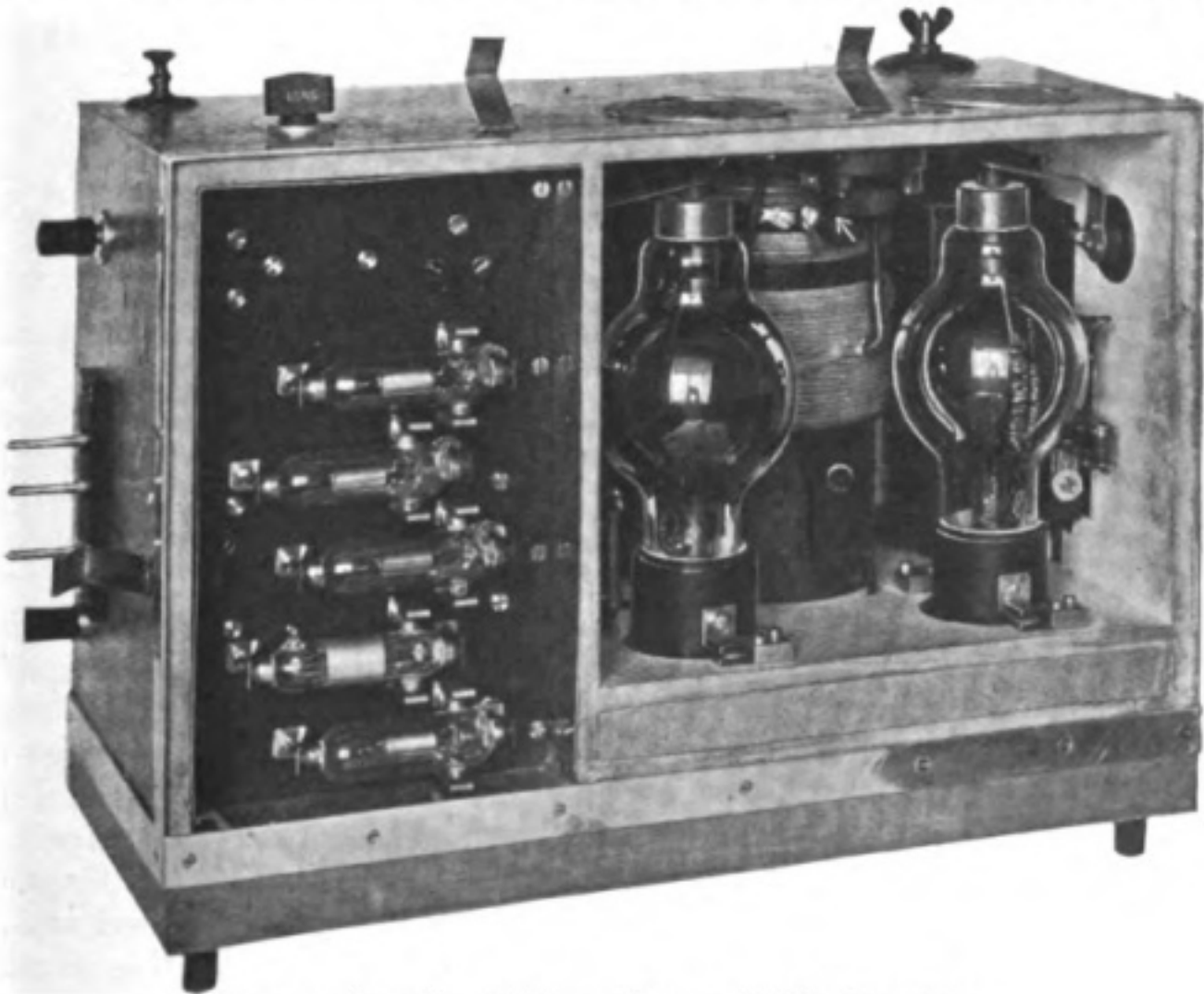
FIG. 2.—Interior of Transmitter and Receiver Box.
