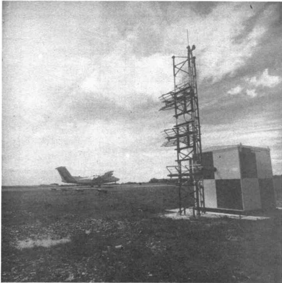
The glide-slope aerial at Plymouth Airport. These are unique in that the approach angle may be switched to either 3 or 7½° (photo: Racal)
