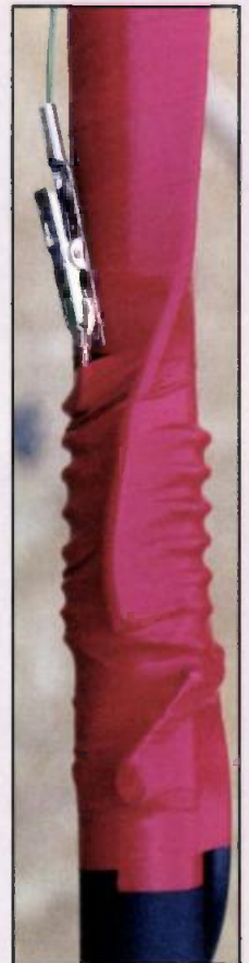
Fig. 6: The final loading coil wrapped up in electrician's insulating tape. The coaxial capacitor runs up the pole under the tape.
