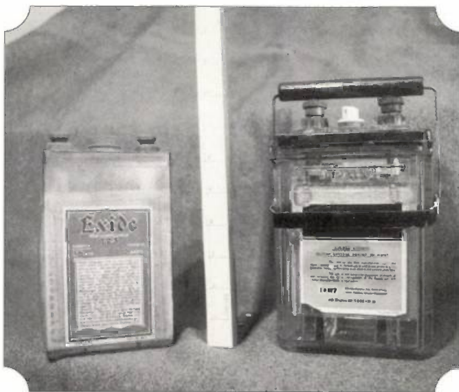
Valve filament supplies were provided by 2V accumulators and many people can remember having to take them to the local garage for 'recharging'. Meanwhile, valve designers were desperately trying to reduce filament current consumption without effecting other characteristics.
