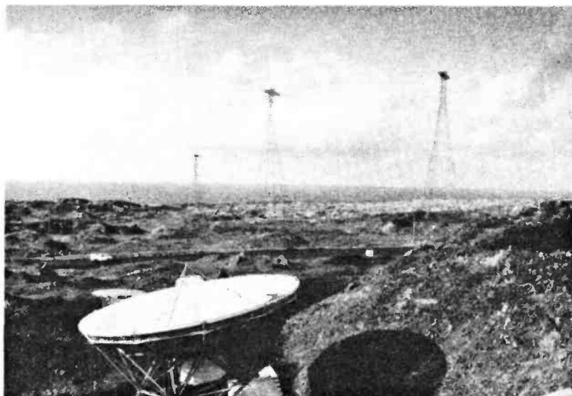
The BBC's Atlantic Relay Station on Ascension Island showing satellite receiving dish for programme feed
