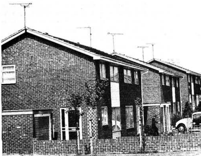
"Various tolerances above the ridge height are informally allowed by authorities from 2m (strong signal area) to 4.5m (in a reception shadow)"
