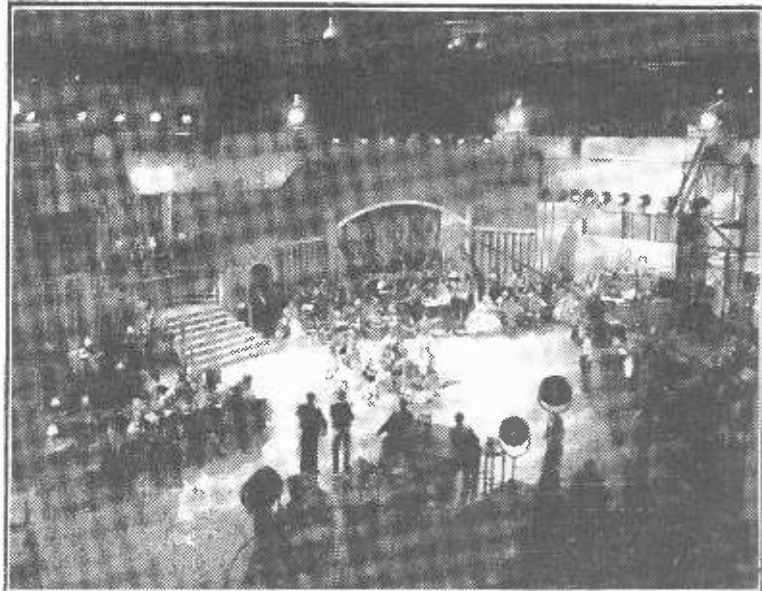
A scene being shot in the B.B.C. studio erected at Olympia for the Radio Exhibition. The studio walls were made of hessian sprayed with cement.
