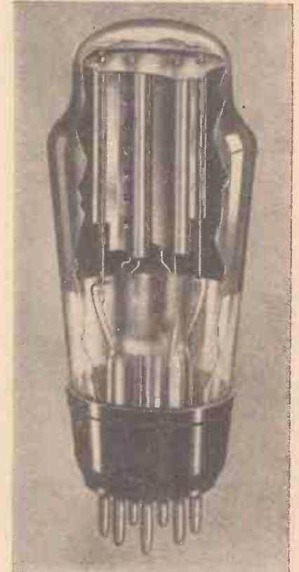
Fig. 3.—A typical Cossor voltage-doubler valve.
